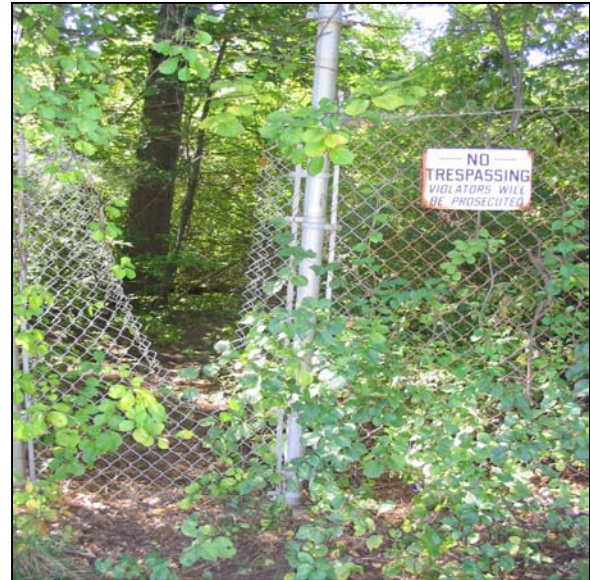
A breach in the fence on Treadwell Street
