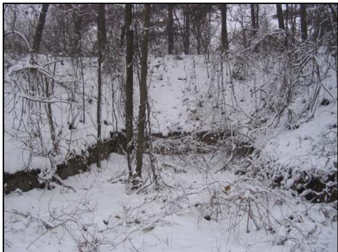
Old retaining wall in the remains of a bunker, which was used by the Winchester Repeating Arms Company for storing gunpowder.
