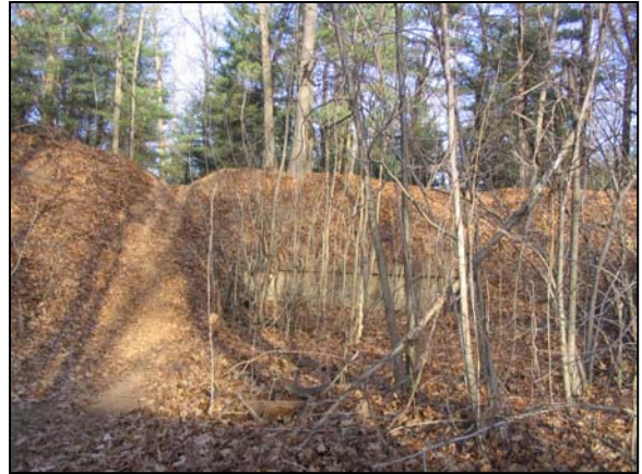
ATV damage, as shown on this bunker, wreaks havoc on the highly erodible soils and steep slopes on the property
