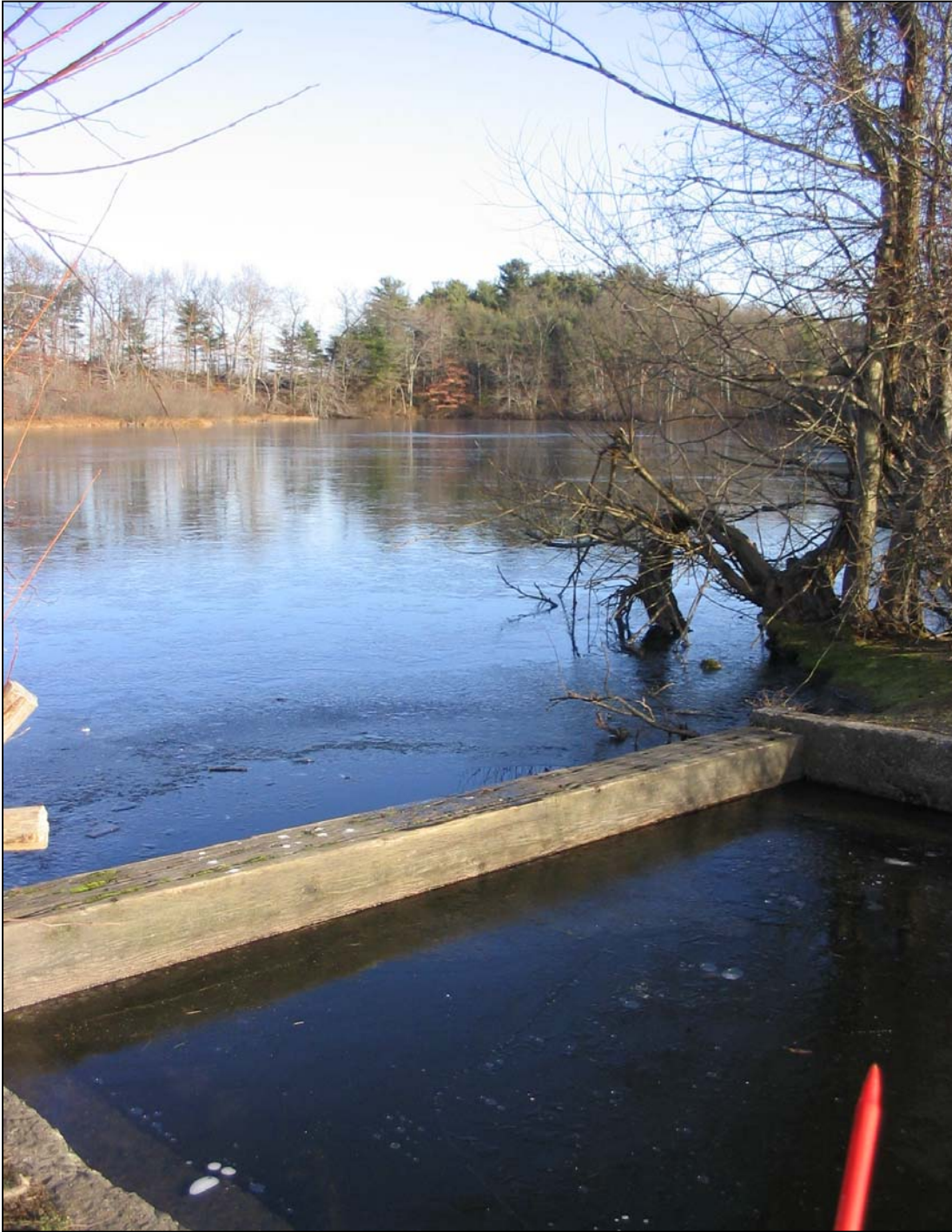
Pond E, view facing northeast, winter 2003
